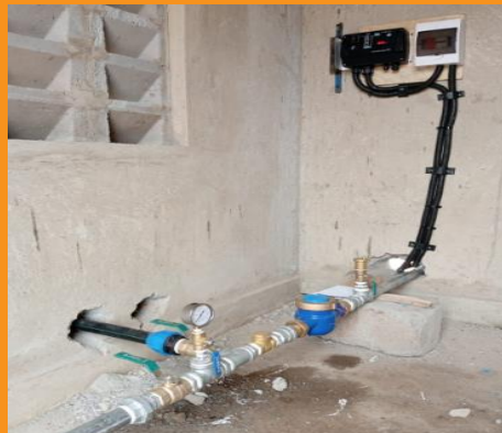
Plumbing works in pump house
