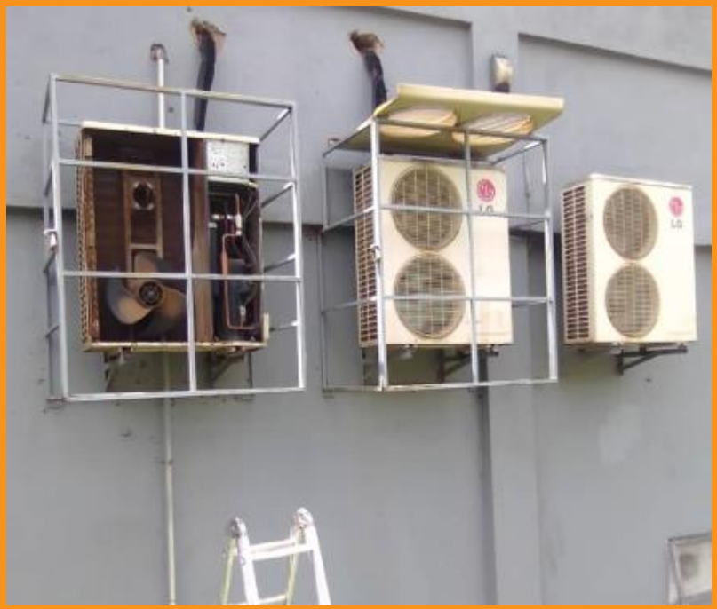
Installation and servicing of AC units of Aseptic lab
