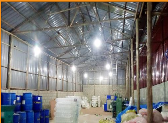
Pet bottle making machine Installation & wiring
